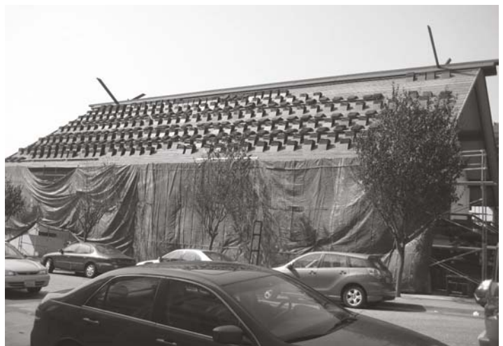
Roof Replacement in progress
